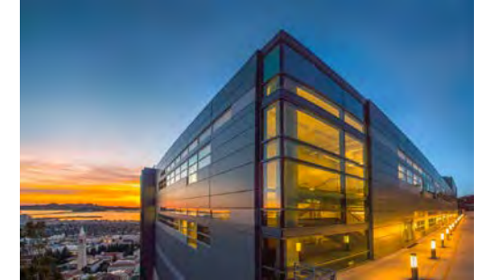
Activate Berkeley at Cyclotron Road
